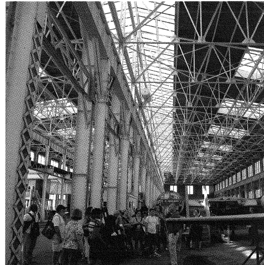
Teachers are dwarfed inside the Back Shop at the North Carolina Transportation Museum. Built in 1905, this building served as the major overhaul facility for steam locomotives. Photo by Lou Nachman.
